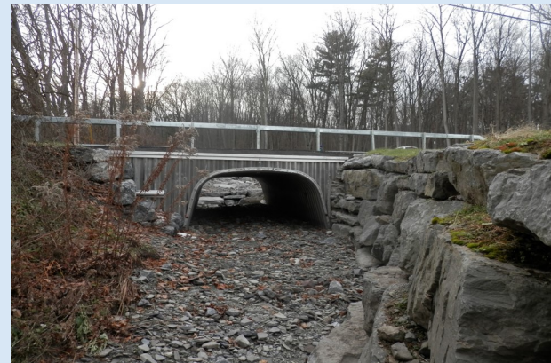
New Arch Culvert Installed
