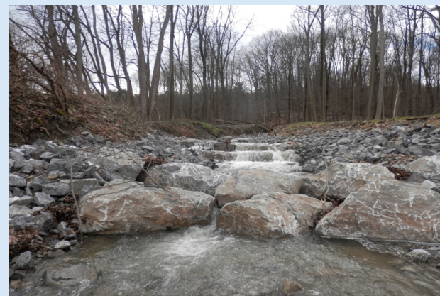
Stream Channel After Grade Stabilization
